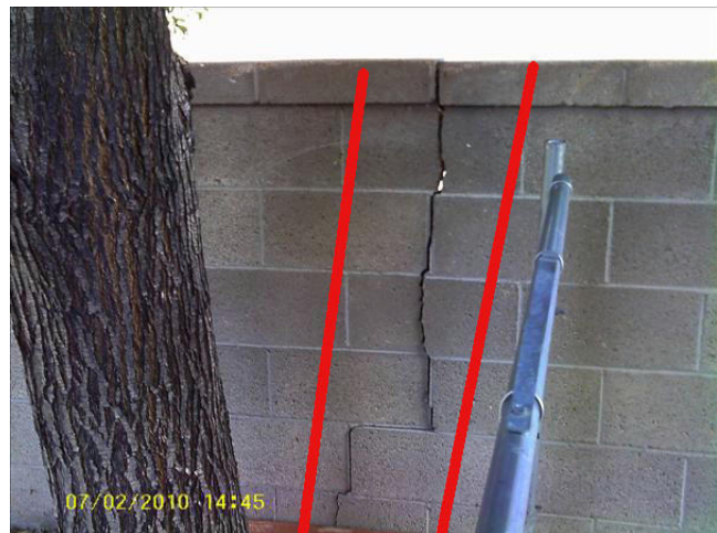
Fence/Gates Fences Maintenance
