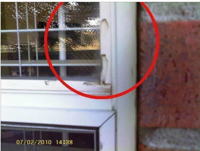
Exterior Structure Glaze/Caulking Window Pane Maintenance
